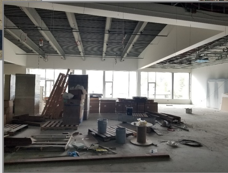
Before and After (+/- 14' and rotated 90 degrees) – Library
