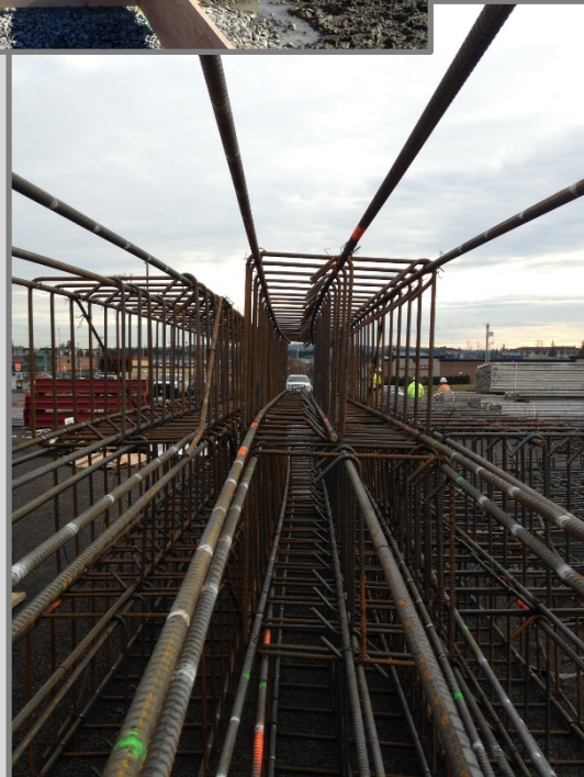
Formwork and reinforcing steel for foundations and walls.
