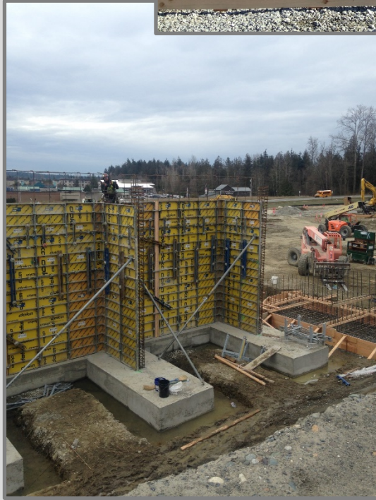
Formwork and reinforcing steel for foundations and walls.
